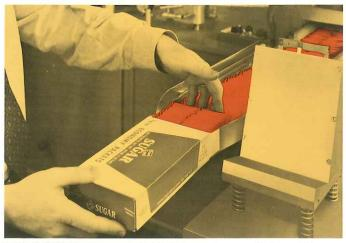
**NEAT STACKER**—Two rows of shingled pouches are discharged from a knife vacuum drop off onto a right angle belt conveyor. The operator inserts a set up box over a loading shoe at the end of the conveyor and identifies the count by a preprinted "alert mark". The packets are manually end loaded and the carton is placed on an adjacent vibrator to settle the load in the carton.
