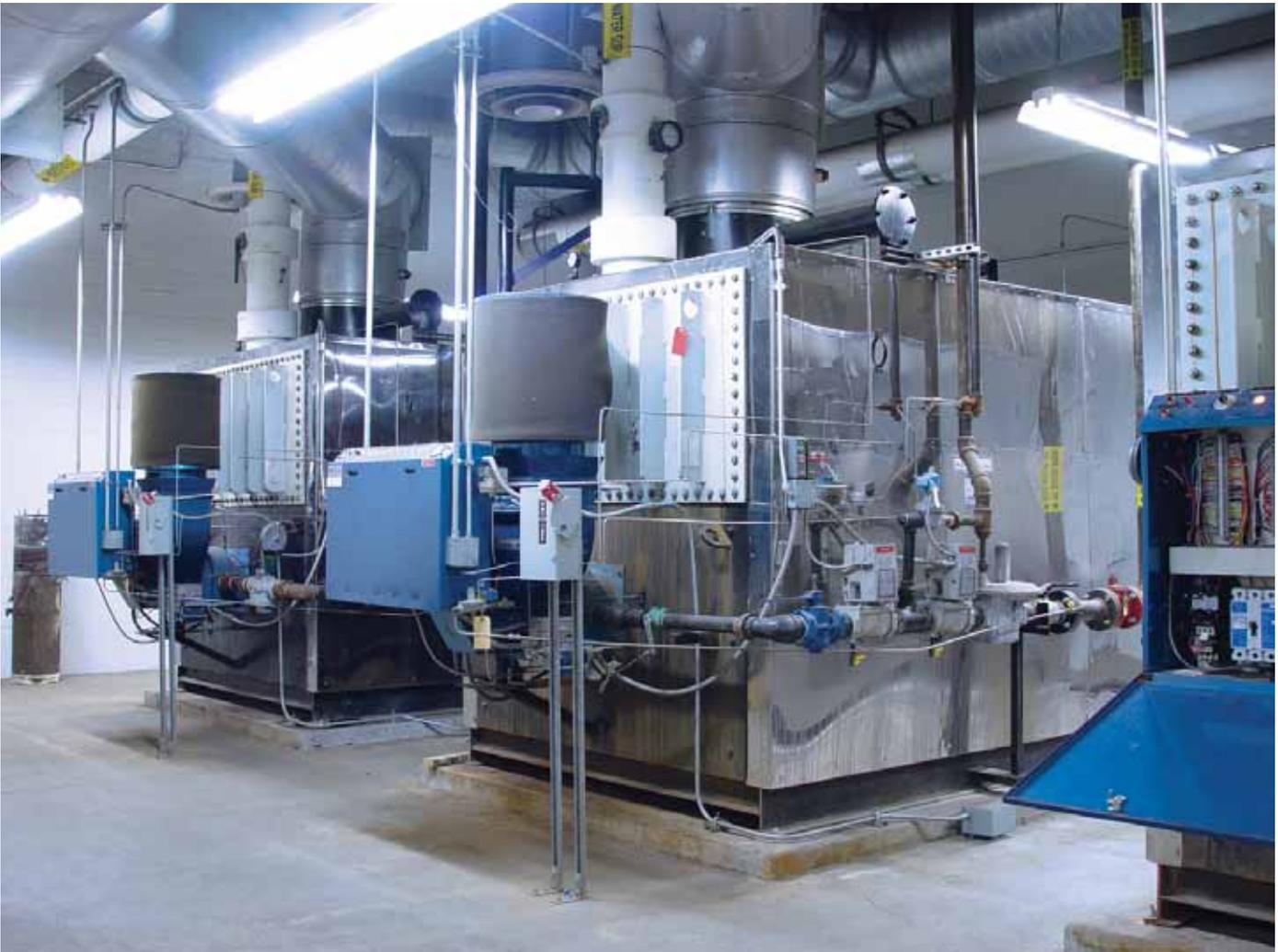
**Solution.** Ajax Boiler supplied three Ajax Series WFG-11500 boilers (11.5 MMBTU/hr per unit). The facility manager uses the three boilers in a lead/lag configuration which gives the convention center the ability to turn boilers on and off to meet varying heat load requirements. Additional benefits include a substantial savings on gas expenses and the ability to shut down a single boiler for service without any interruption in heat for convention center attendees.
