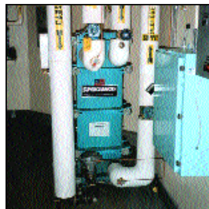
SUPERCHANGER heat exchangers recover heat very efficiently because of their high heat transfer rates and close temperature approach capabilities.
