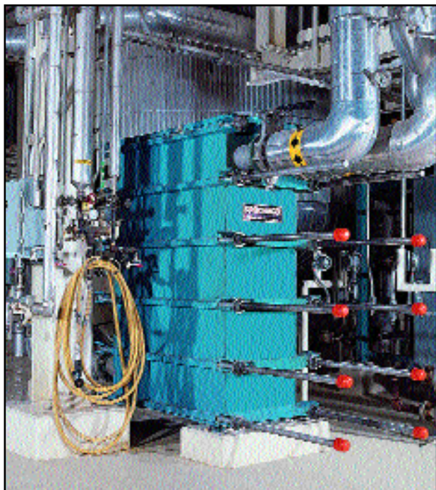
Pictured here is a SUPERCHANGER heat exchanger performing one of hundreds of duties in the food processing industry, which include process heating or cooling (many with viscous fluids), basic water heating and heat recovery from waste streams.
