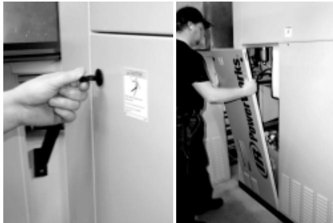
*Figure 39. Removing the left rear enclosure panel*
