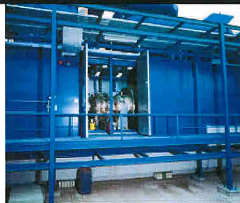
Institutional Cogeneration Mars 100 Turbine Generator Set, Tri-Fuel Paper Plant, Turkey
